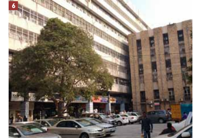
Parking Lot 6 : Surface parking in Lok Nayak Bhawan complex open to public. Basement parking is reserved for employees in the complex.
